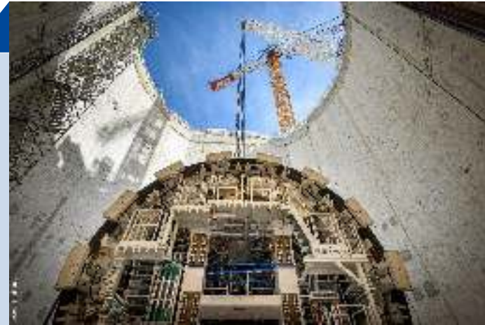
Lowering of the Caroline TBM's cutter head in Massy
