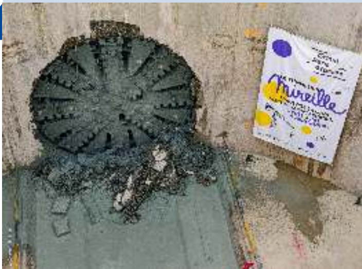
Breakthrough of the Mireille TBM in Clichy-Montfermeil
