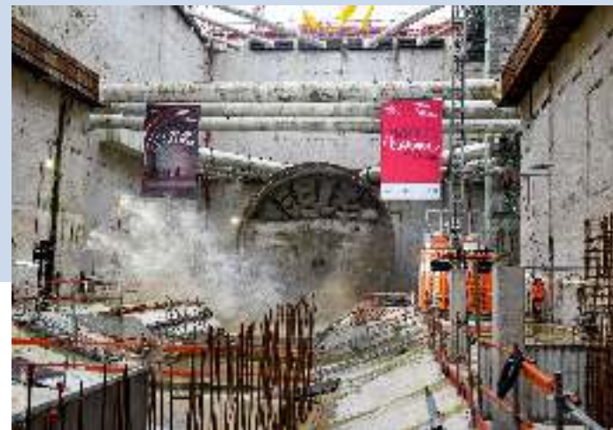
Breakthrough of the Marina TBM in Créteil l'Echat
