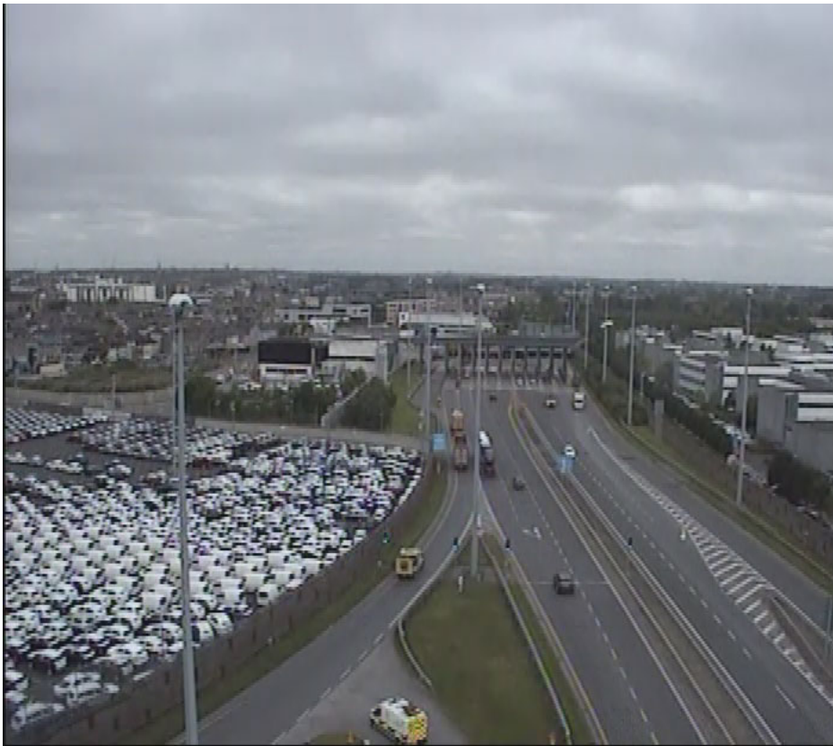
Port Tunnel Entrance / East Wall Dublin City CCTV 26 Jun 2019 10:07:34 GMT Daylight Time
