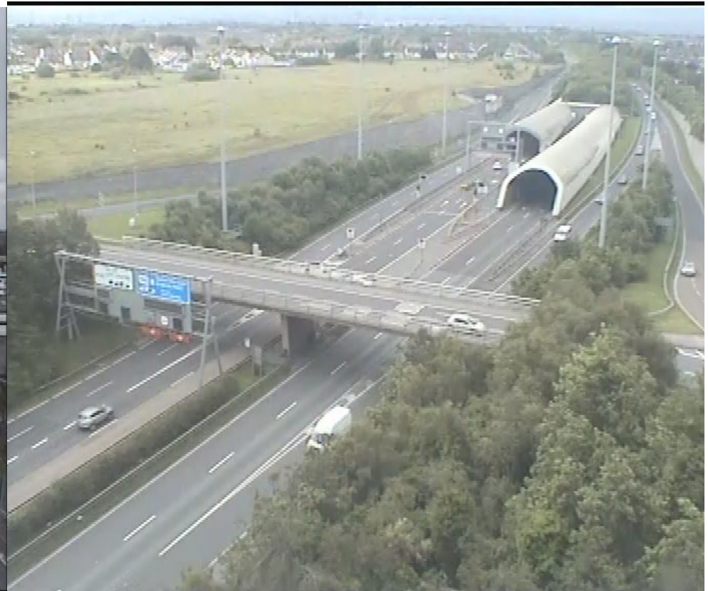
M50 / Coolock Lane Dublin City CCTV 26 Jun 2019 10:09:37 GMT Daylight Time
