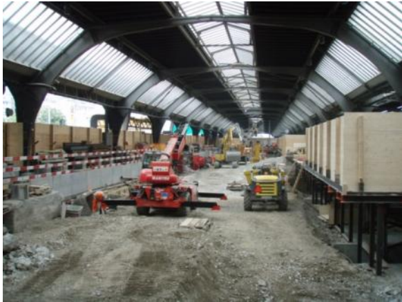
Cross-City Train Line, construction work in the Zurich Main Station
